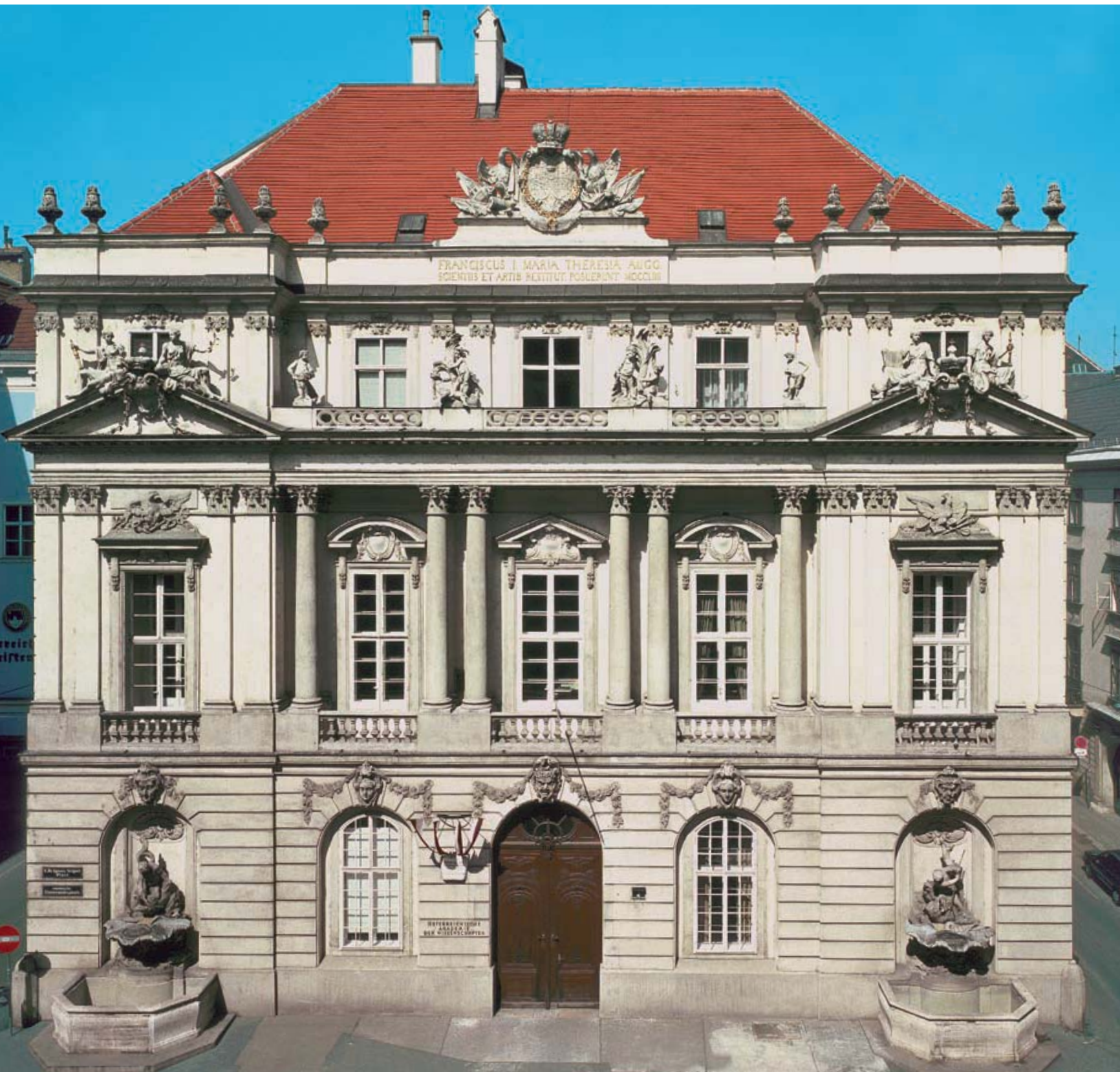
ACADEMY BUILDING, PRINCIPAL FAÇADE (FIG. 21)
